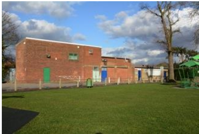
Current community building
